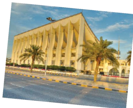
Focus on: The National Assembly Building
